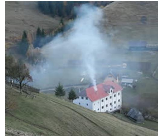
Old house with a boiler
