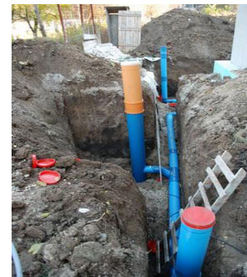
Condensation tower of the EAHX
